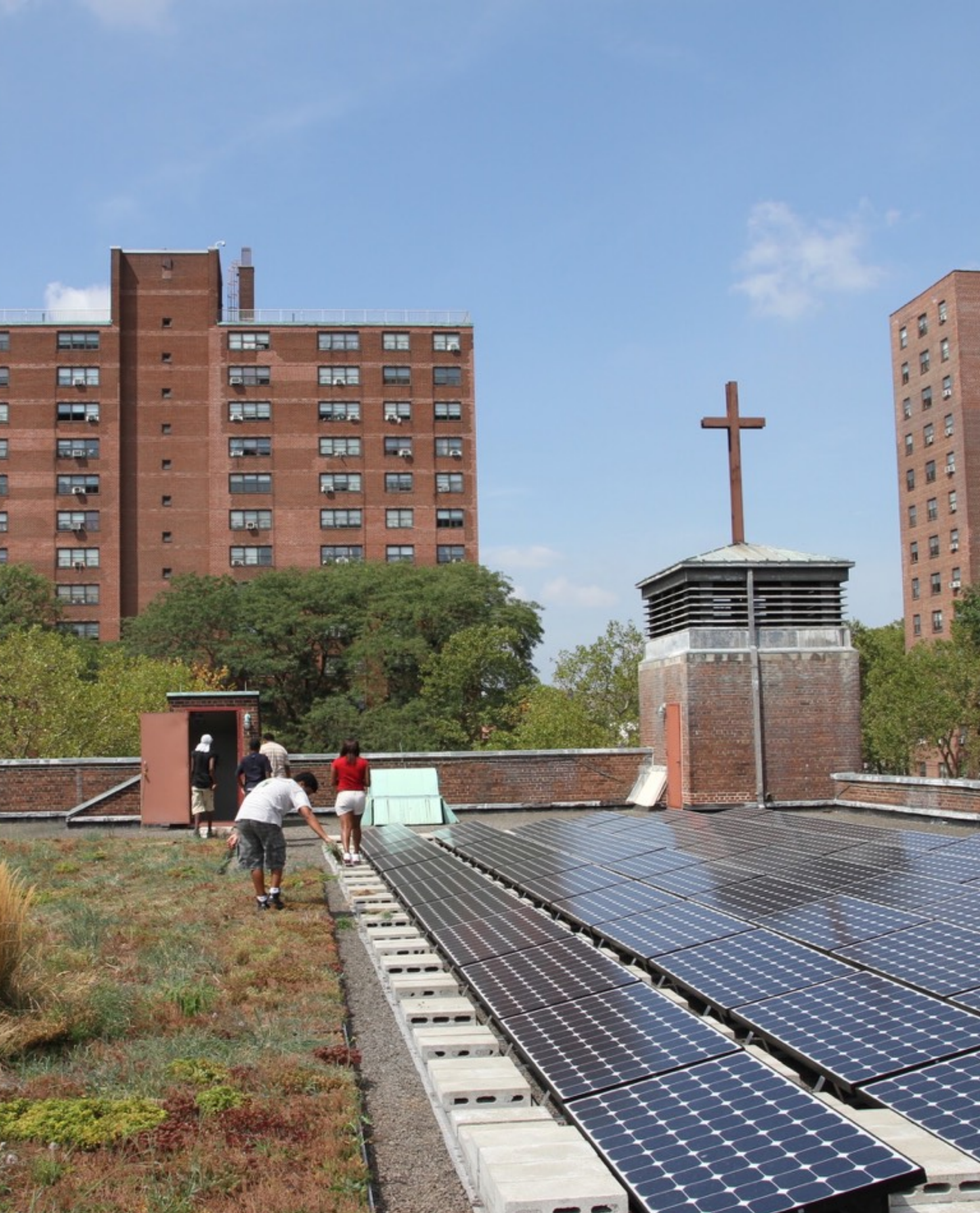
Green roof on top of St. Joan of Arc church in the South Bronx.
