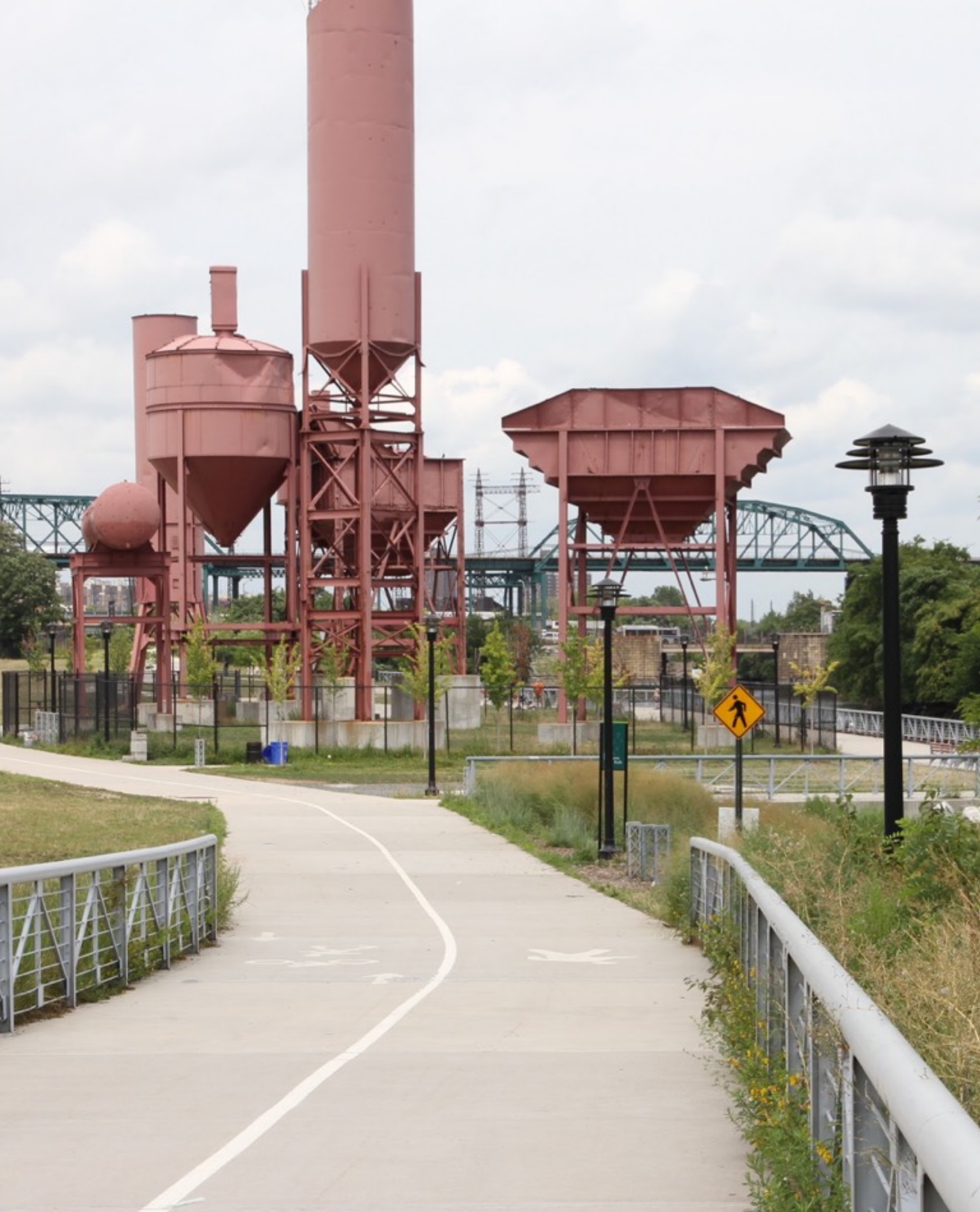
Concrete Plant Park, a public part in the South Bronx, was created by the Parks Department in partnership with community-based organizations.
