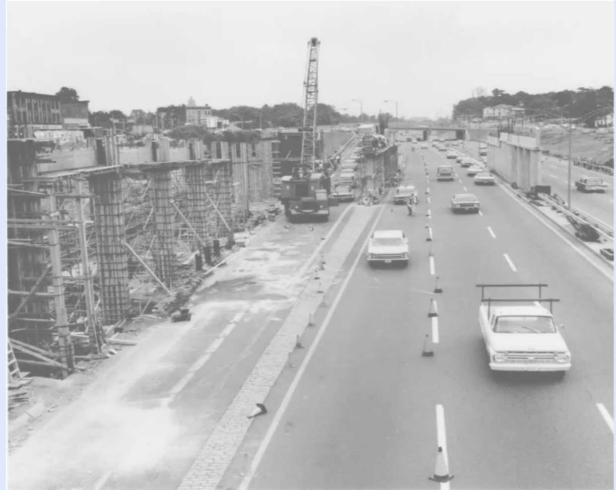
Image of the MA Pike being built through West Newton, MA
