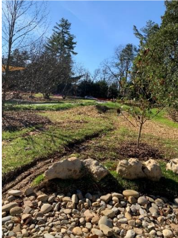
Figure 3: Another view of berms that were created to assist flow of water.
