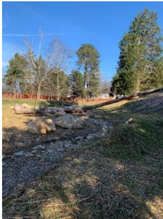
Figure 2: Compacted rocks and dirt, or berms, were added to initial stream after observing flow of water.
